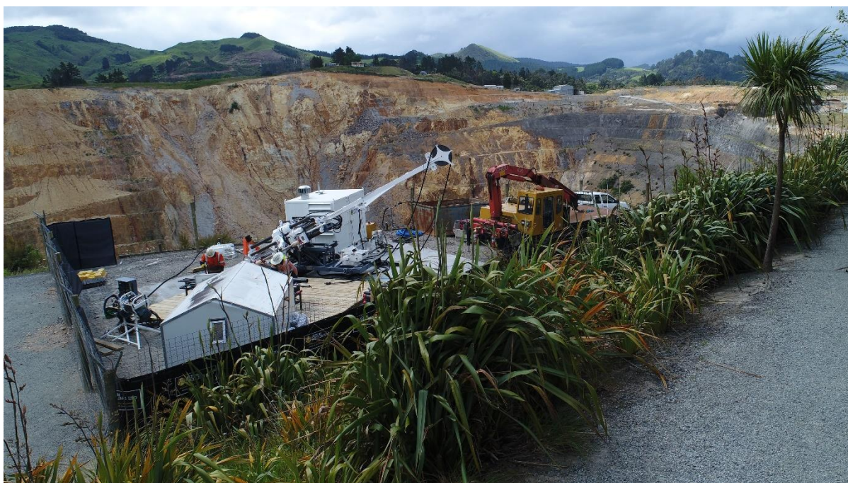
Martha Underground resource drilling at the Waihi Operation.
