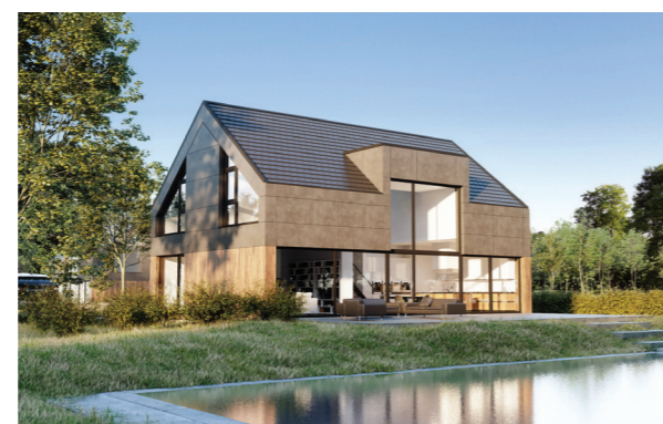
Module building of Danwood S.A., which has been taken over by GS E&C
