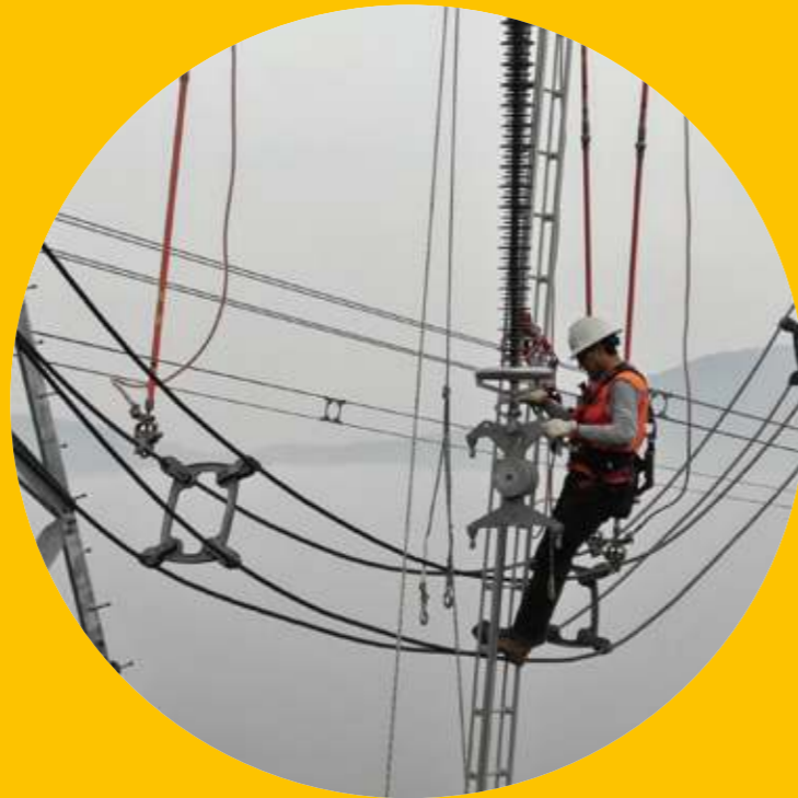
Anti-climbing system being installed by Maule maintenance team.
