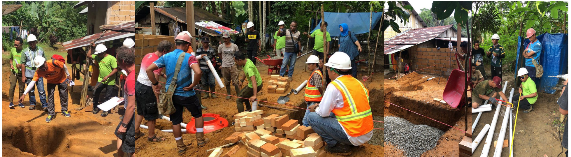
GAR installing SWGs in Indonesia
