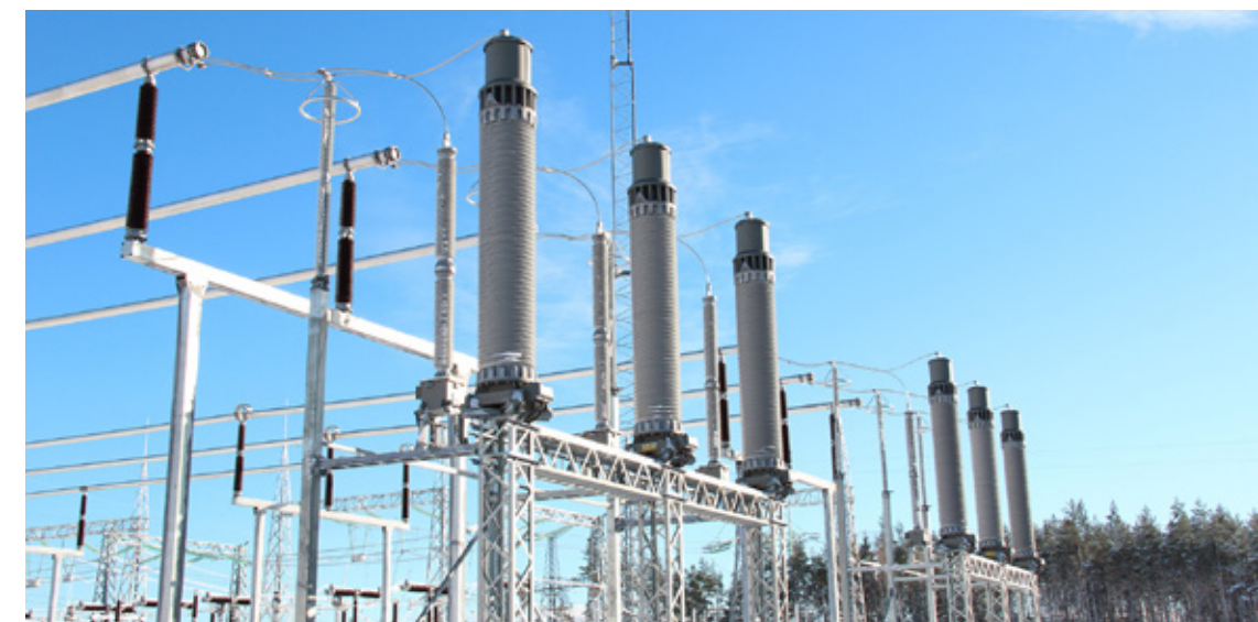
KONČAR 362 kV high power voltage transformers
