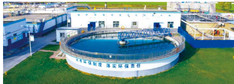
Sewage treatment plants
