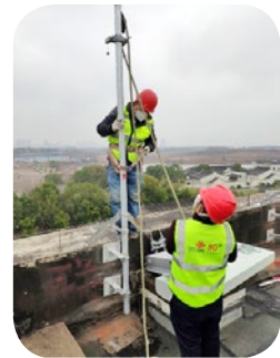
Construction site of communications network for Huoshenshan Hospital
