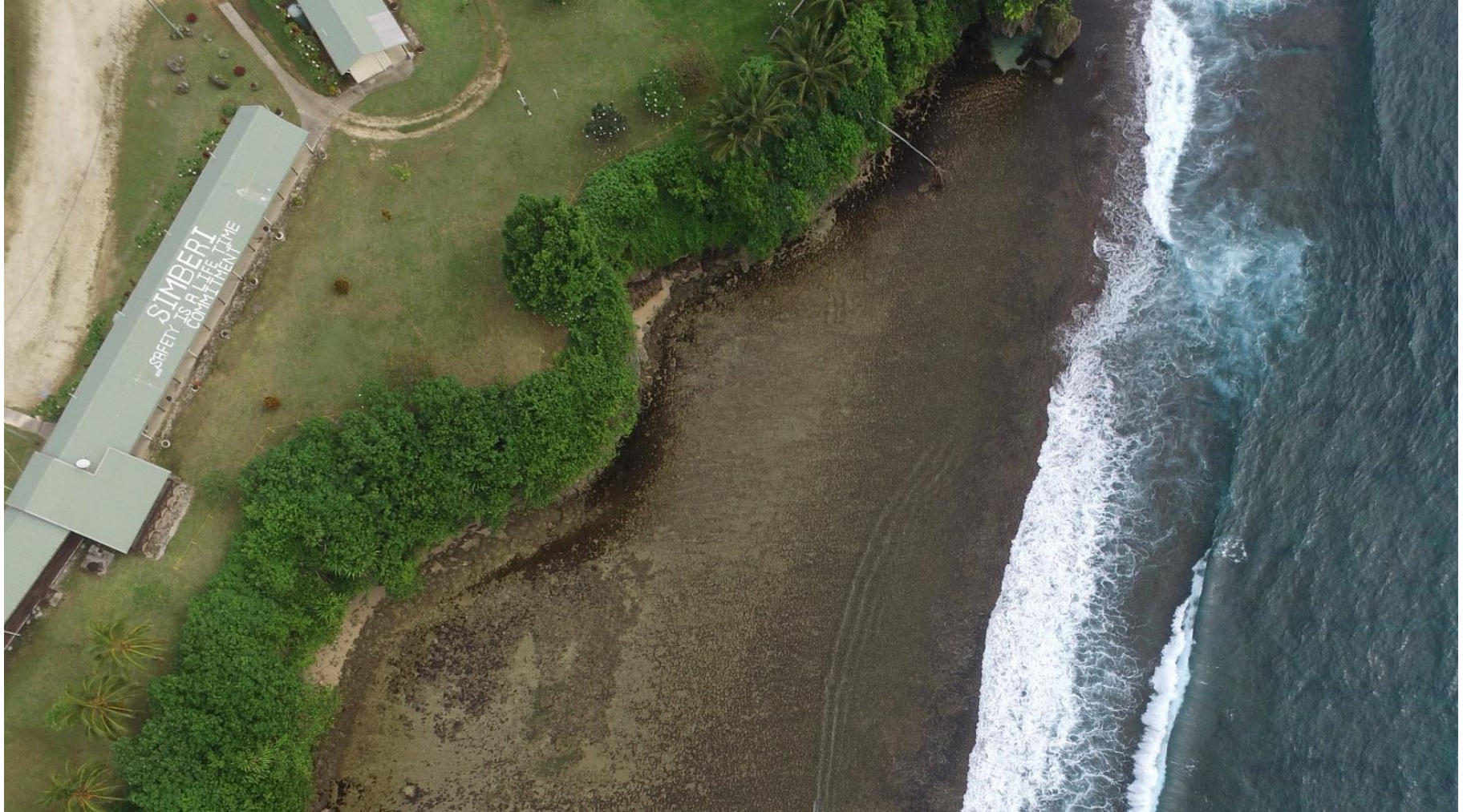
Photo: 'Simberi- Safety is a life time commitment' – painted on the roof of accommodation block F at Simberi camp. Photo by Ivan Andrew via drone.
