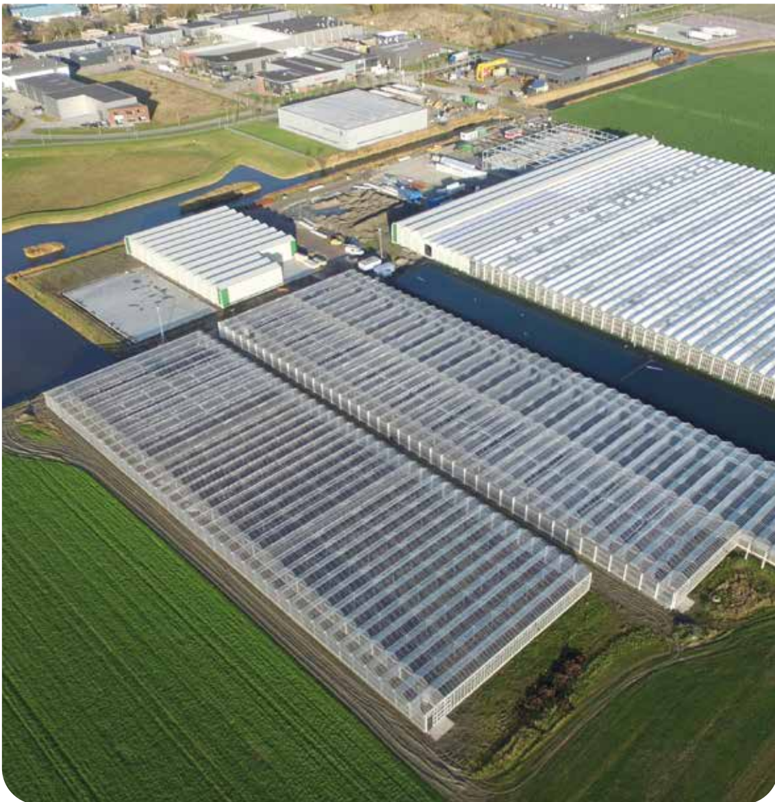
Hazera – Warmenhuizen site (Netherlands): construction of this new research station is set to boost performance in terms of water and energy.
