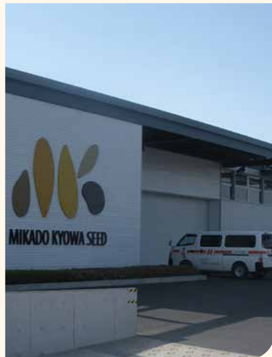
Vilmorin Mikado – Toké site (Japan): the company has introduced liquefied natural gas into its energy mix, thereby reducing its greenhouse gas emissions
