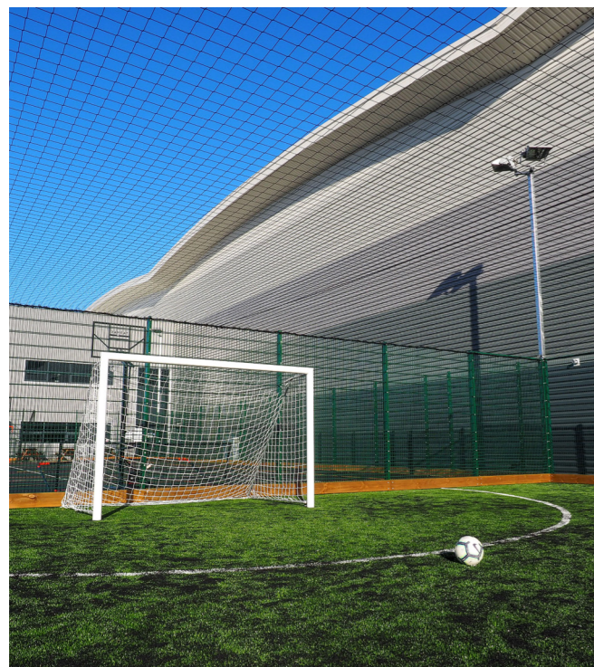
Decathlon platform, Northampton (United-Kingdom)
