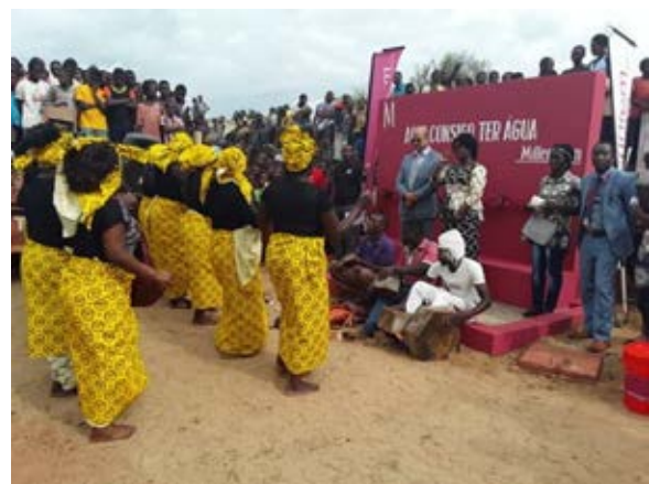
Installation of a fountain in the village of Namialo (Nampula), improving access to drinking water (Mozambique)
