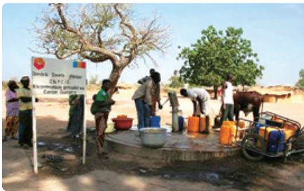
Water well drilling for Gudawa
