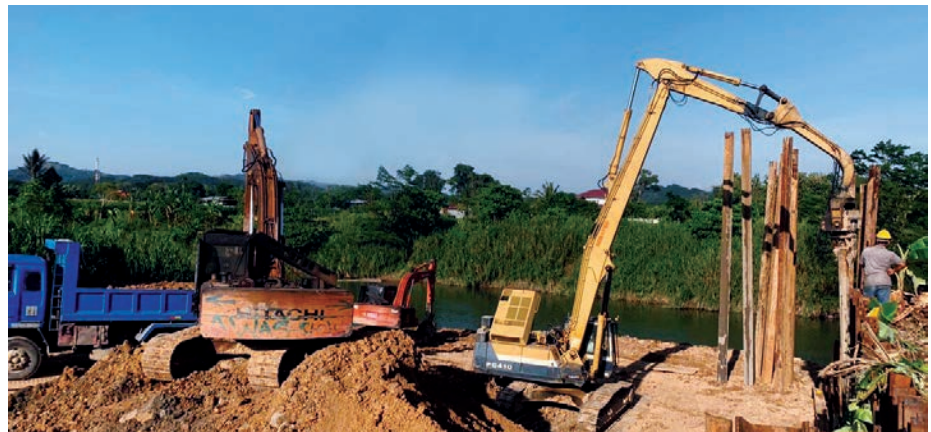
▲ Construction of Telibong II Water Treatment Plant in Sabah
