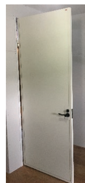
Cardboard door in accommodation blocks
