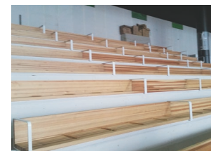
Timber temporary seat model (January 2019)
