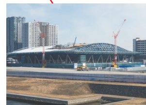
Use of timber roofing (January 2019)
