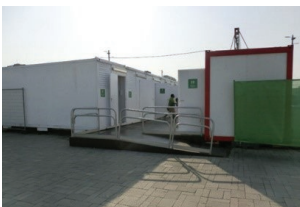
Example of Modular toilets
