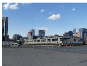
Tsukiji Transportation Depot under construction (as of February 2020)
