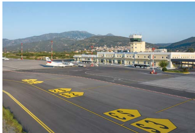
Construction work on the Samos airport in Greece was completed on time.
