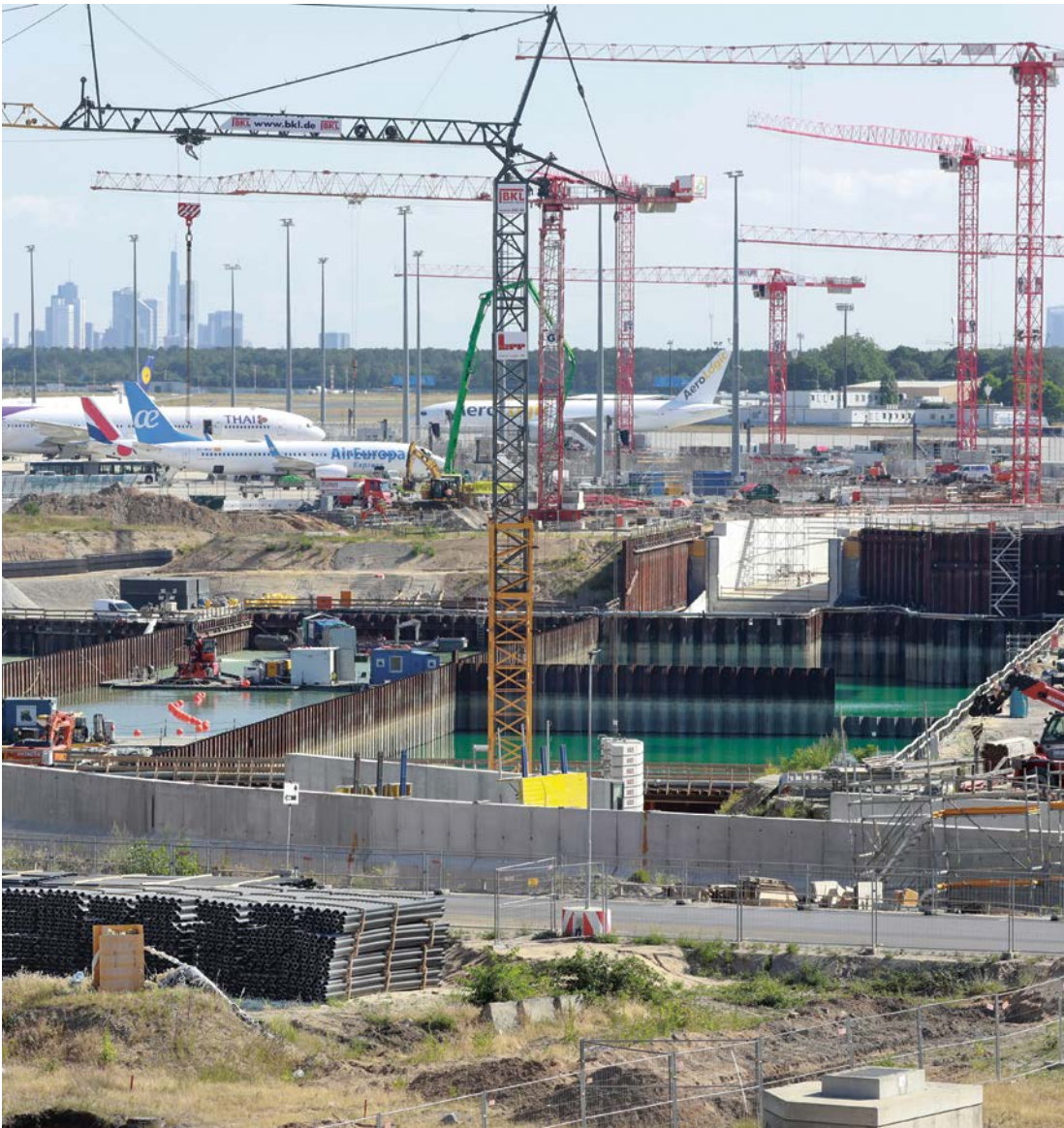
Major construction site Terminal 3 in the southern part of Frankfurt Airport
