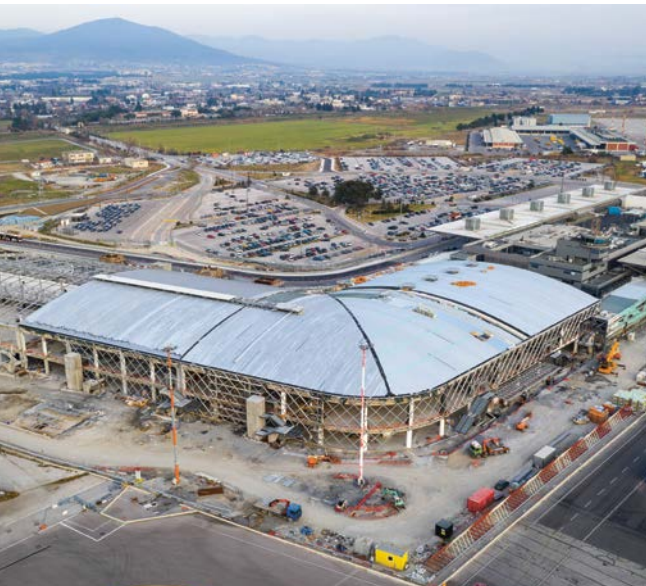
A new terminal is being built in Thessaloniki for around €100 million.
