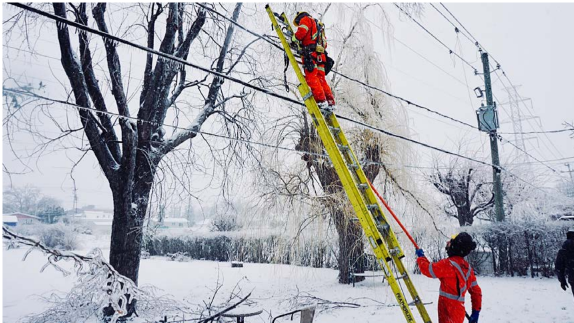
Line crew repairing the damage caused by freezing rain in April 2019.
