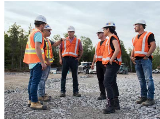
Employees at the Achigan substation jobsite.
