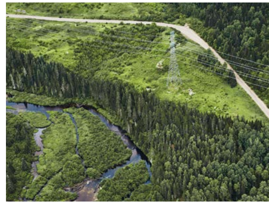
Segment of the 735-kV Micoua-Saguenay line.
