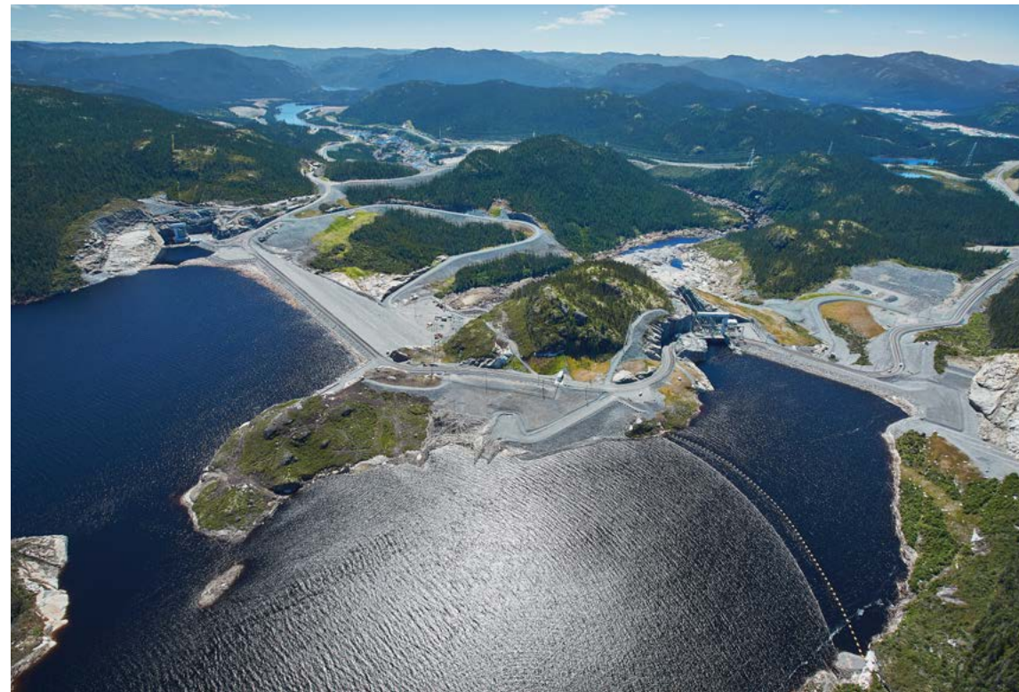
Romaine-3 generating station, commissioned in 2017.
