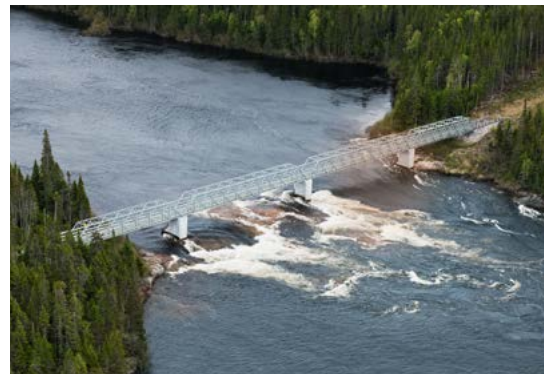
A snowmobile bridge at Romaine-1.
