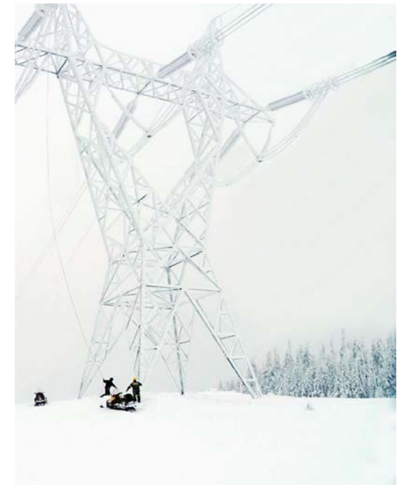
Ground-wire repair on the Saguenay-Jacques-Cartier line.
