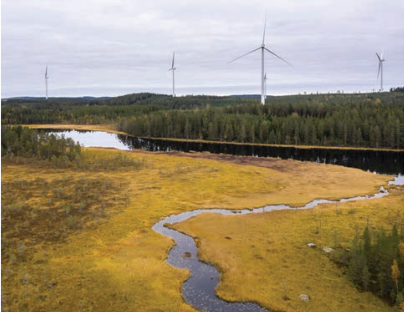
Consideration for valuable countryside at Valhalla wind farm (366 MW) in Sweden. Photo: Joakim Lagercrantz
