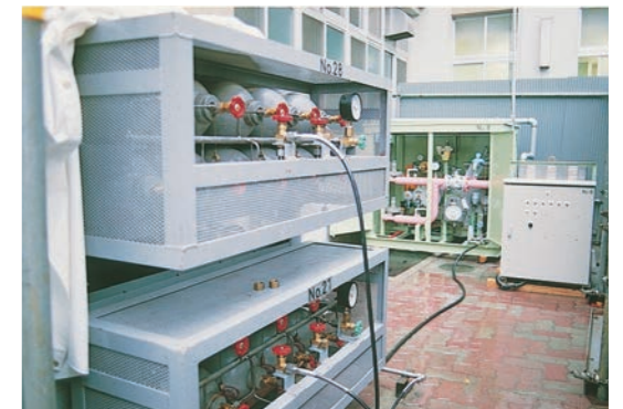
Portable gas generator (top) and temporary bath facilities, powered by CNG (FCV), installed following the Great Hanshin-Awaji Earthquake
