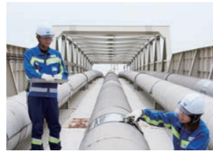
Regular inspection of bridge piping
