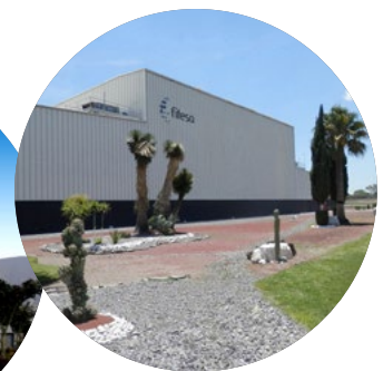
Front view of Fitesa in Mexico, San Jose Iturbide.
