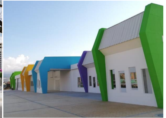
Colegio Torrente – Soacha,
