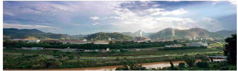
Aperam Timóteo plant, in the Brazilian "Steel Valley" in Minas Gerais.
