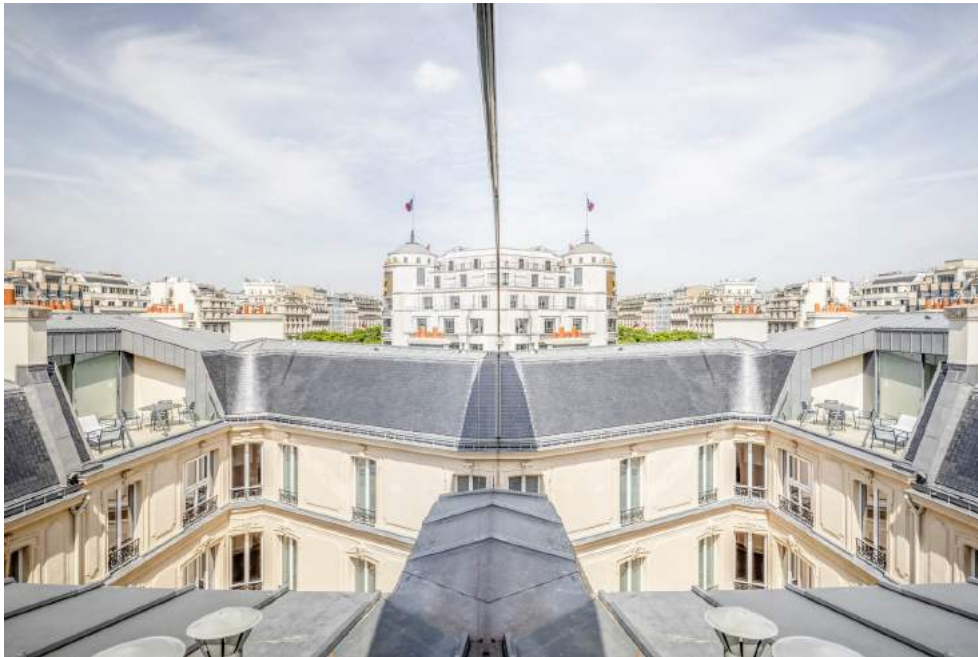
Caption: Fouquet's - Agence Vous êtes ici Architectes / VEI © 11h45 / Florent Michel Executed using grade Aperam 316L with Uginox Meca 8ND (super mirror finish) A recent renovation has restored the building to its original state. In addition to refurbishing the guest rooms and amenity areas, the project also reworked the interior courtyard. To hide the ventilation ducts that run through the space, architects added an 18 m high, 10 m wide stainless steel wall that essentially serves as a screen. Adding a contemporary aesthetic to the landscape, the material's mirror finish increases natural light and reflects the opposite façade, giving the impression that the courtyard is more spacious than it really is.
