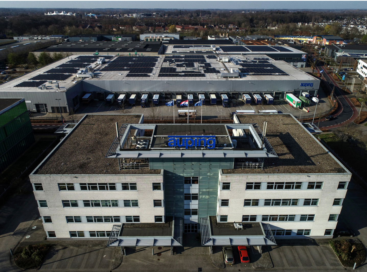
Headquarters and production Auping, Maagdenburgstraat Deventer, the Netherlands
