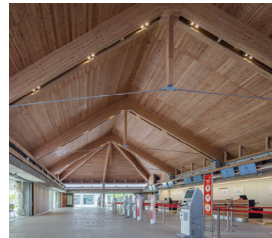
Check in lobby using CLT as structural material for the roof
