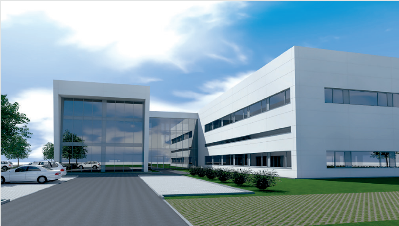
The new HEINE company building in Gilching (planning photo): On the left the 3-storey administration building, on the right the production building.
