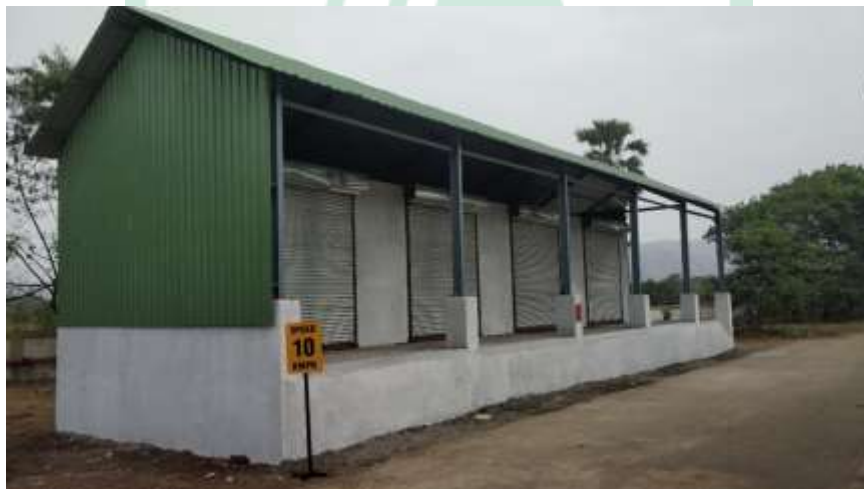
Separate area for hazardous waste storage at IP – Taloja
