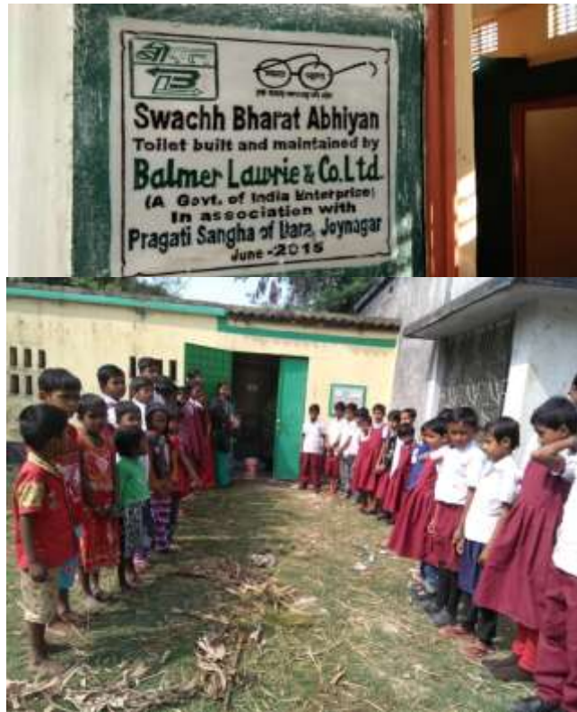
Toilet maintenance in a Government school in West Bengal
