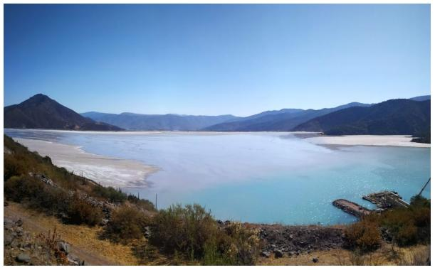
The El Torito tailings dam at El Soldado Mine, Chile: water reclaim pond and barges, wet beach and sand wall in the distance.
