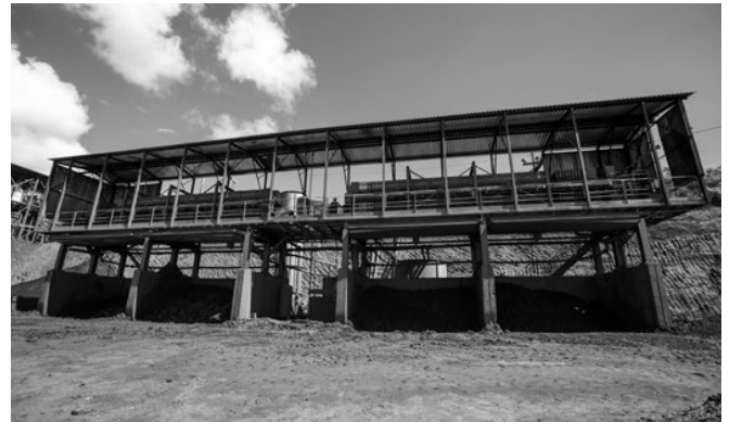
Installation of press filters
