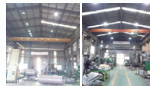
Before & After Installing High-efficiency Lighting Devices for Suppliers
