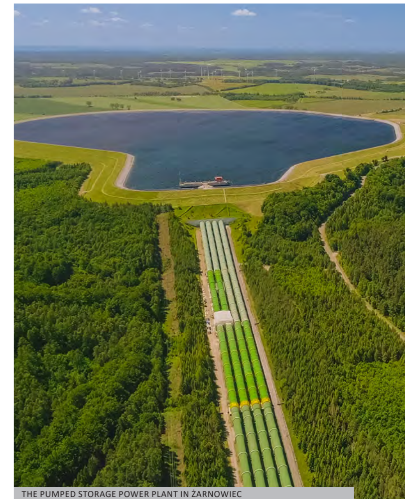
THE PUMPED STORAGE POWER PLANT IN ŻARNOWIEC
