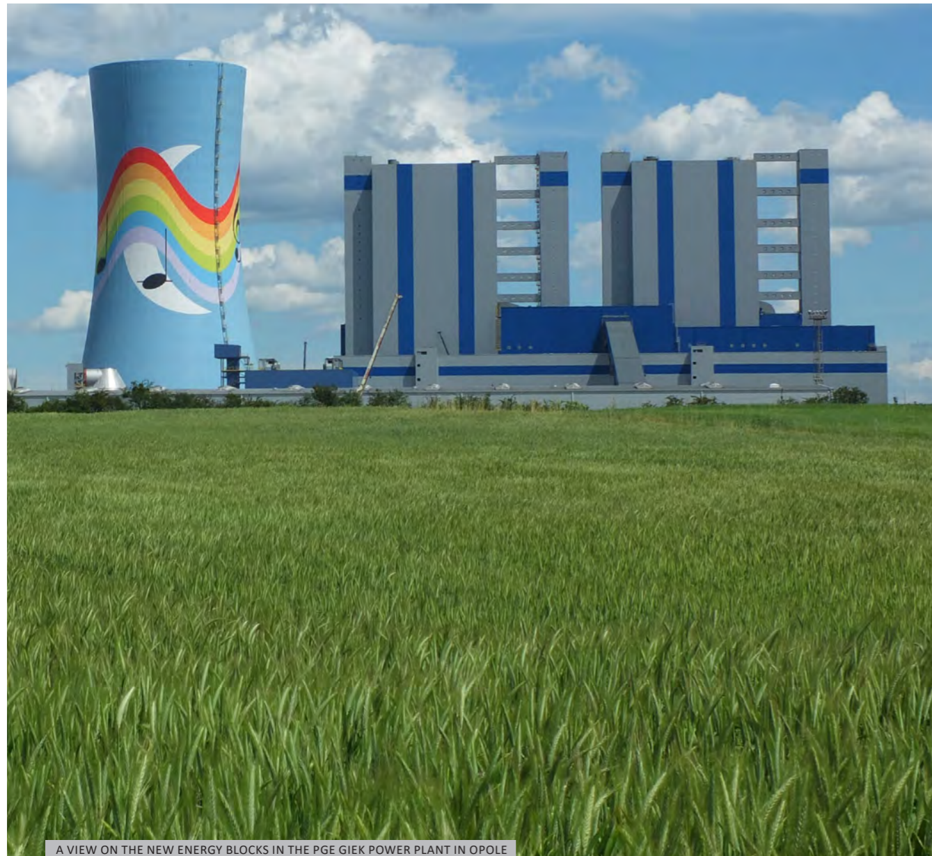
A VIEW ON THE NEW ENERGY BLOCKS IN THE PGE GIEK POWER PLANT IN OPOLE
