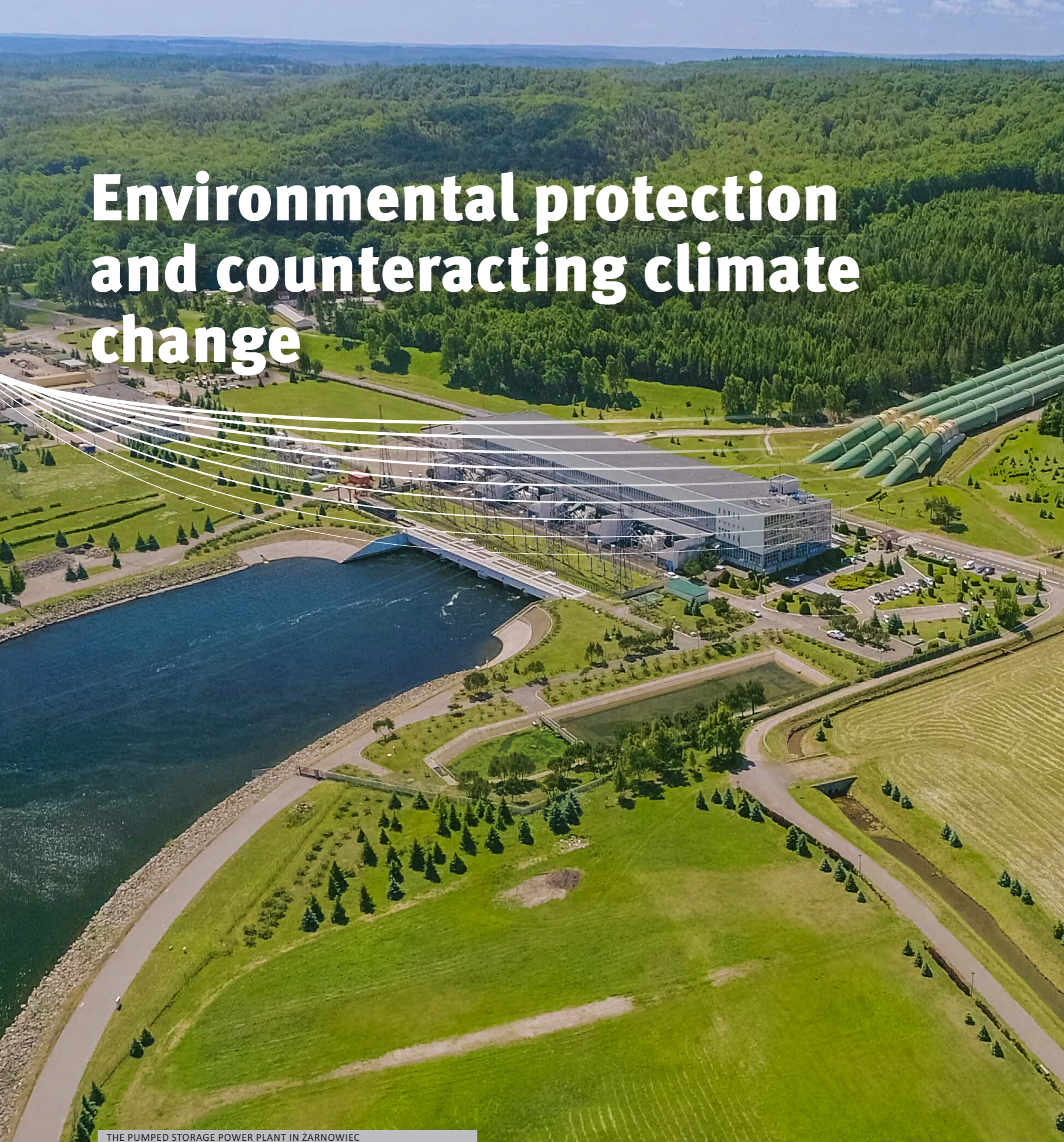
THE PUMPED STORAGE POWER PLANT IN ŻARNOWIEC
