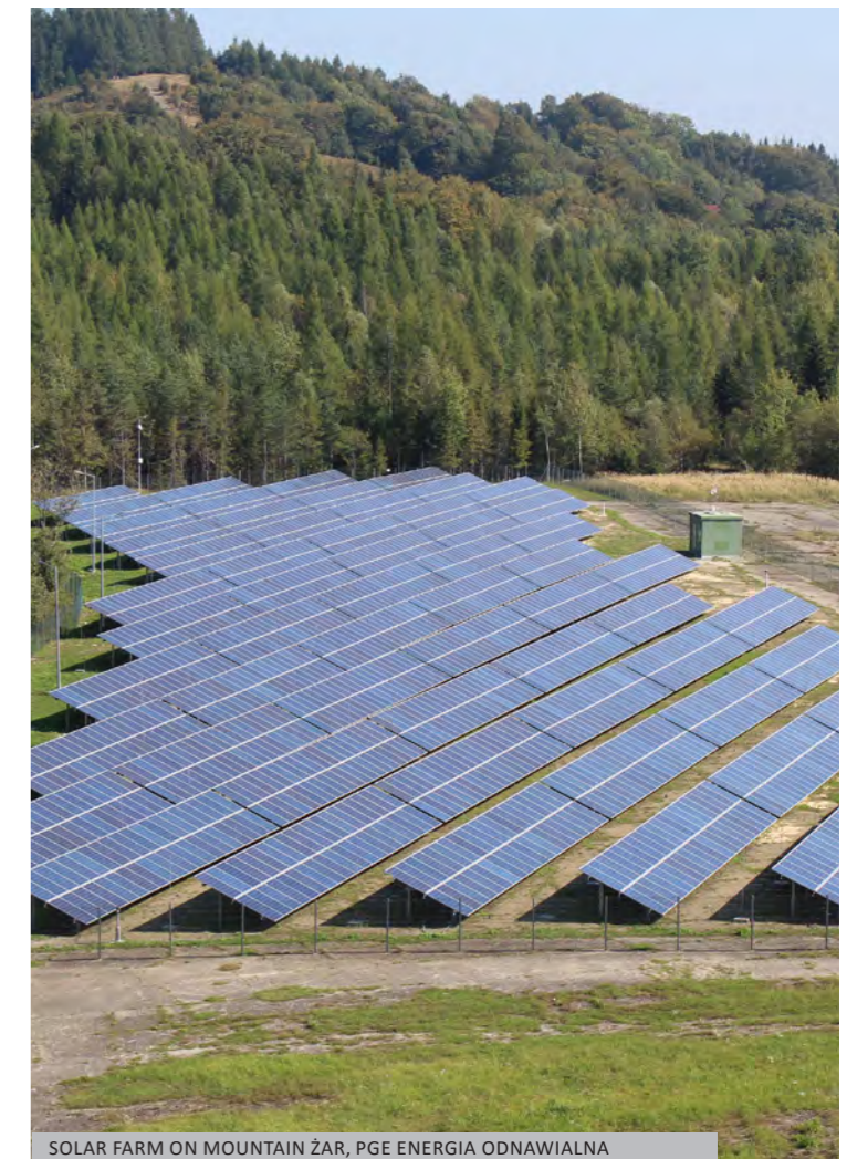
SOLAR FARM ON MOUNTAIN ŻAR, PGE ENERGIA ODNAWIALNA
