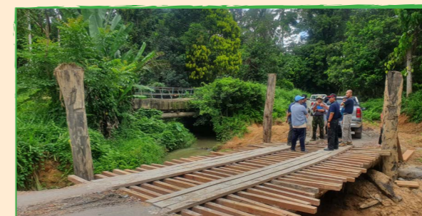
Temporary bridge in the foreground taken in August 2019
