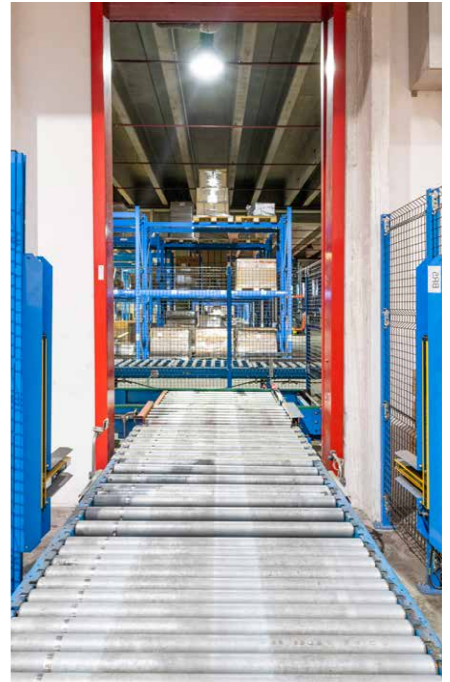
Automatic Shipping Warehouse - Artemide Factory Pregnana Milanese
