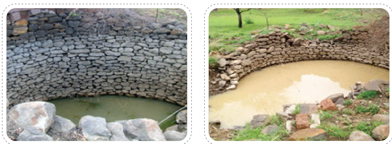
Showing a clear rise in water level in a dug well post treatment work during the monsoon season compared to the water level before treatment
