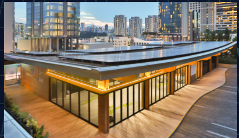
South Beach's microclimatic canopy covered with PV panels (top picture). Singapore Sustainability Academy (SSA) is a zero-energy and BCA Green Mark Platinum building opened in June 2017 (bottom picture).
