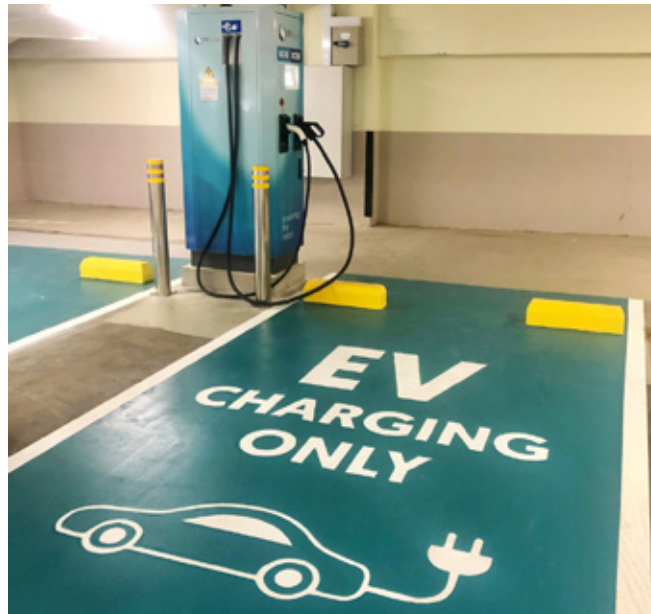
In partnership with SP Group, the direct current fast chargers at Republic Plaza can charge a car in 30 mins, bringing greater convenience to EV drivers in the CBD.
