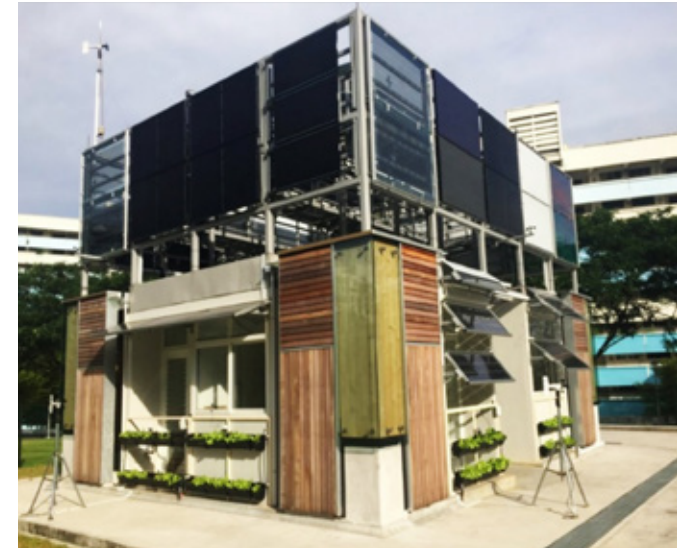
Through running trials such as the integration of solar panels and fast-growing farming systems into the NUS-CDL T 2 Lab’s modular building façades, the Lab studies the impact on natural cross ventilation, daylight, and thermal comfort in buildings.
