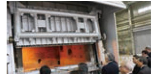
Aluminium continuous casting facility introduced at Kanbara Works
