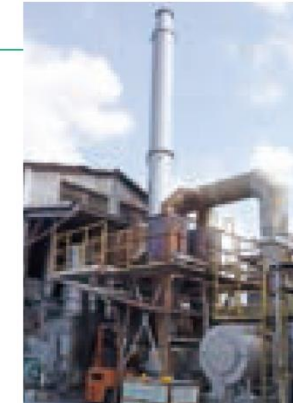
Dismantled incinerator at the Yao Works
