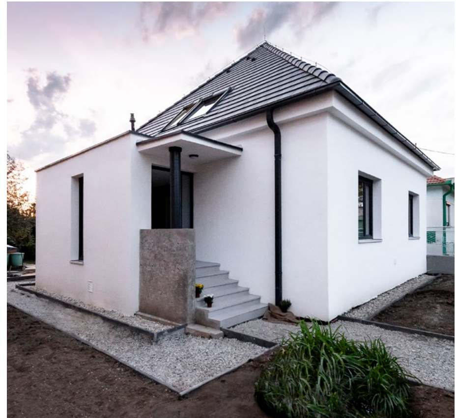
The home after renovation
