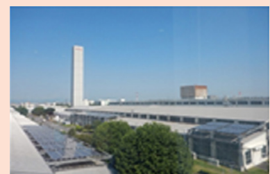
Fuchu Complex is promoting introduction of photovoltaic power generation and high-efficiency production facilities
