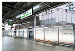
Hydrogen-based Autonomous Energy Supply System H2One™
