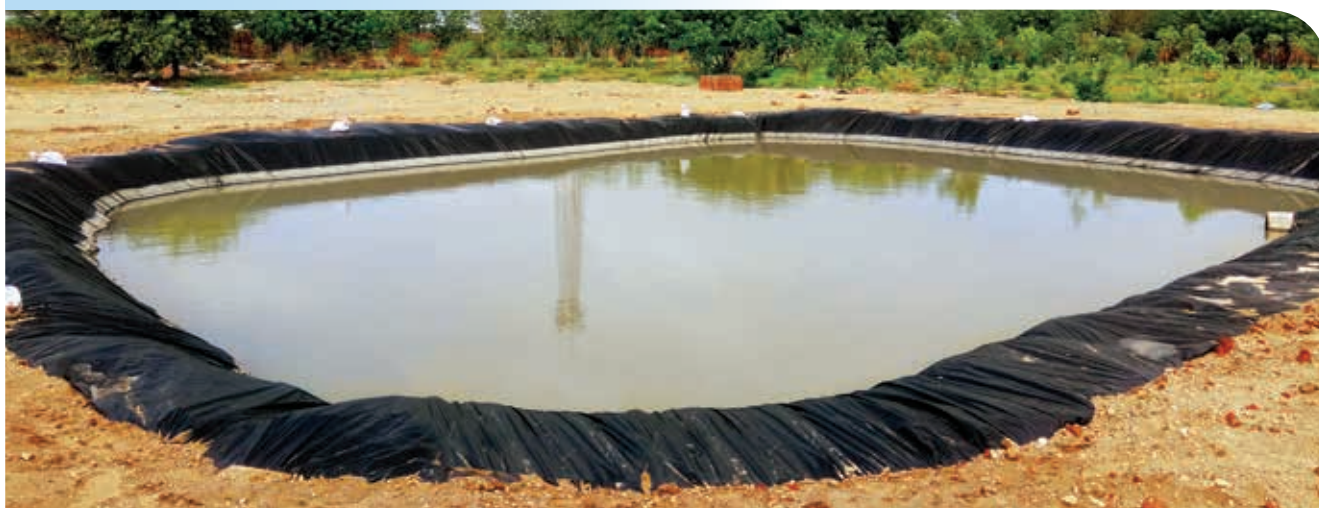
Rainwater collection pond at Jodhpur IRD
