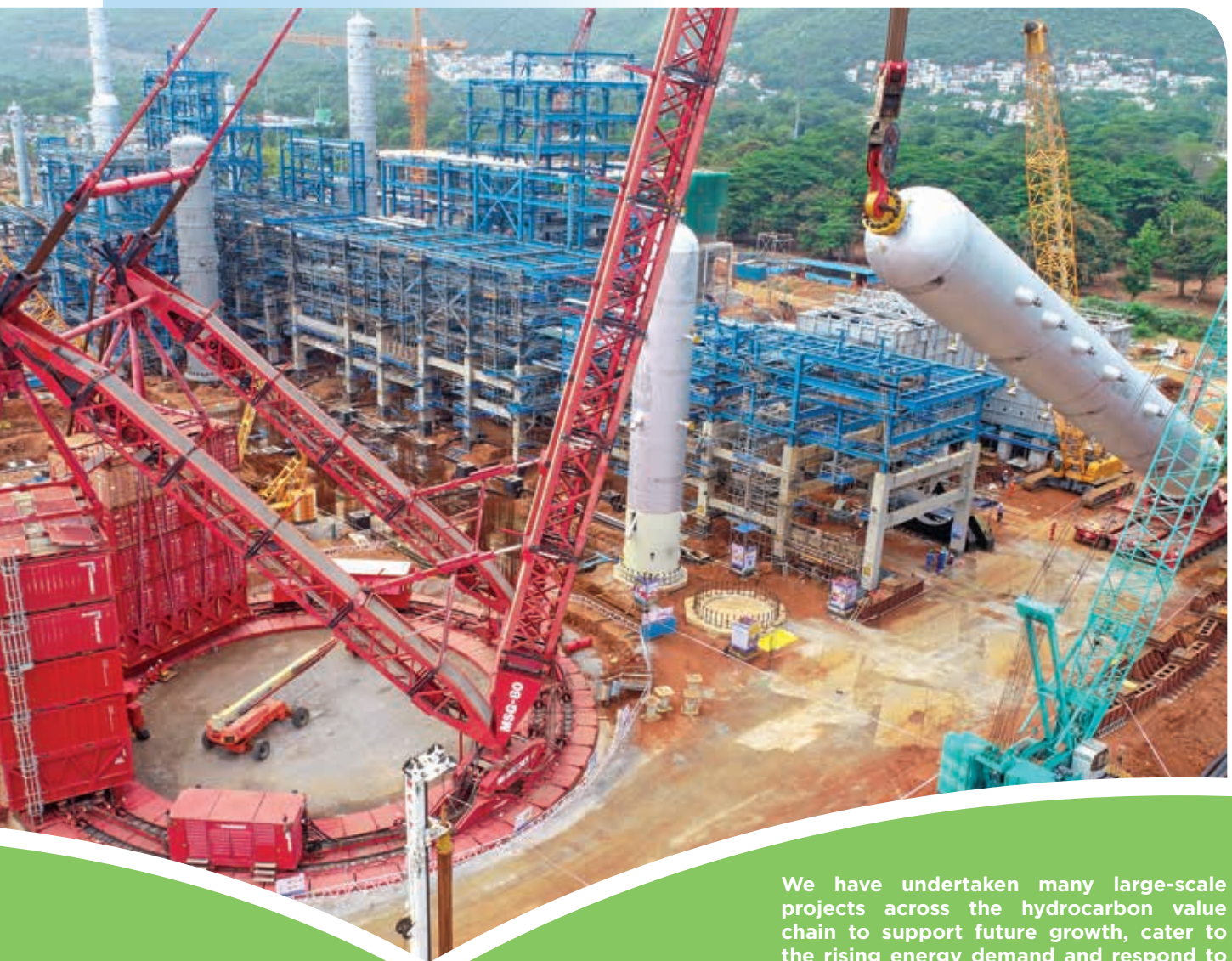
Visakh Refinery Modernisation Project
