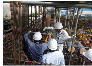
A quality control inspection at a construction site
