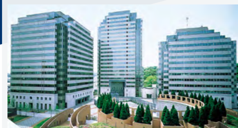
1988 Starts construction of Yokohama Business Park (YBP), one of the largest business park developments conducted solely by the private sector
