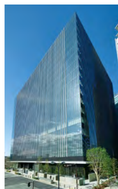
Yokohama Nomura Building
