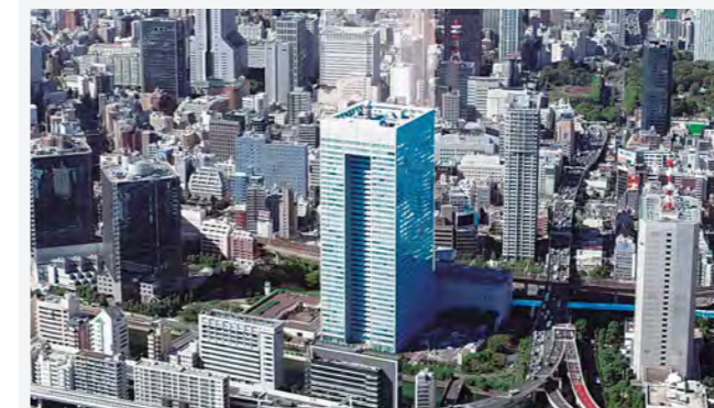
2008 NREG TOSHIBA BUILDING Co., Ltd. joins the Nomura Real Estate Group
