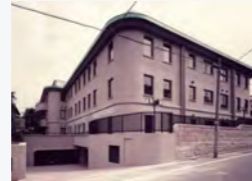
PROUD Uehara Forest Existing property completed in 1984
