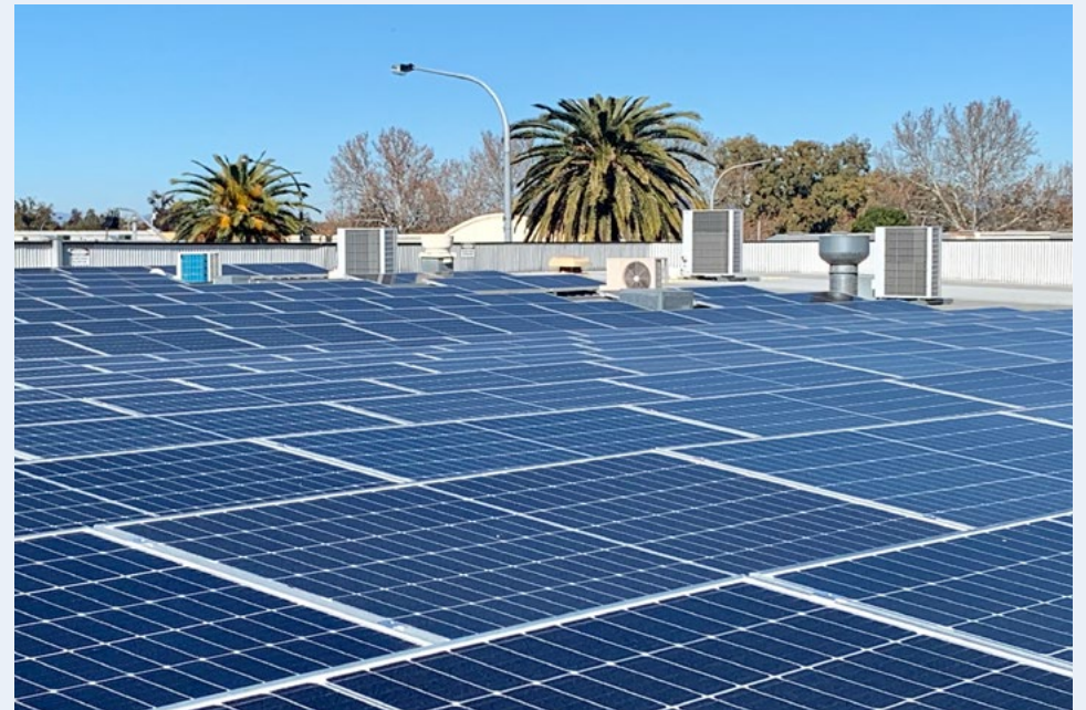
Tamworth Square, Tamworth NSW
