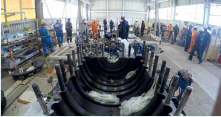
Maintenance during turnaround 2018.
