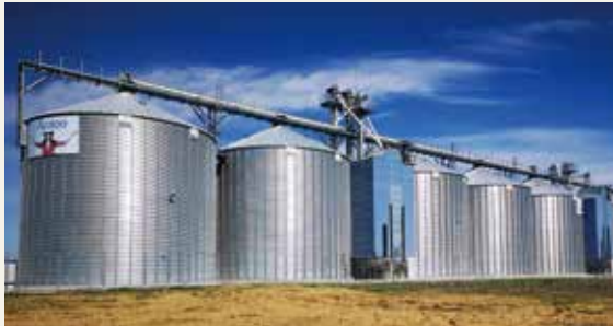
Alcedo's grain silos in Romania
