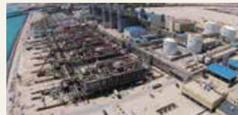
Az-Zour North 1 Independent Water Power Producer (IWPP) project, Kuwait
