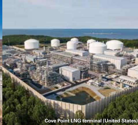
Cove Point LNG terminal (United States)
