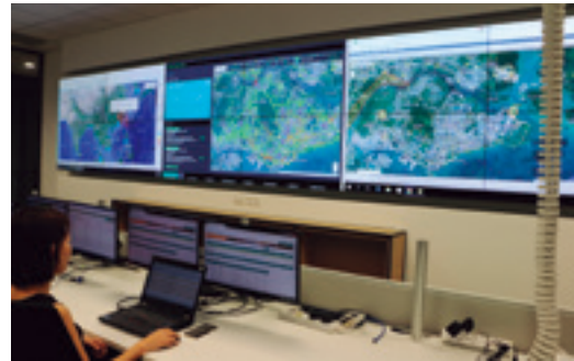
SiTadeL Control Tower for vehicle operation throughout Singapore
