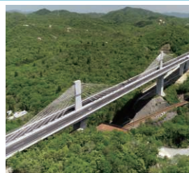
Construction Work of the Shinmeishin Expressway Ikuno-ohashi Bridge (PC upper part Work) (Kobe-shi, Hyogo)
