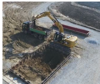
Automatically controlled digging and loading processes
