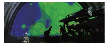
Ground information projected onto the tunnel face
