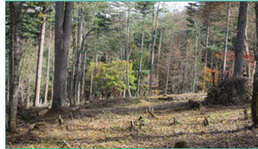
▶ Ground clearing complete
