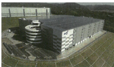
Solar power panels at MFLP Ibaraki (generation capacity approx. 2,000 kW)
