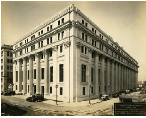
The new Mitsui Main Building (Chuo-ku, Tokyo)
