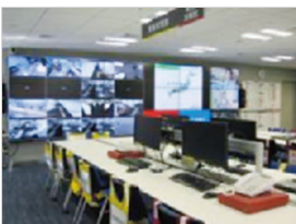
Disaster Countermeasure Headquarters (Mitsui Building No. 2)
