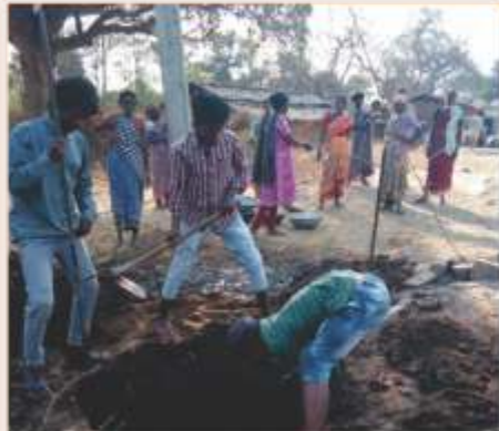
Construction of Soak-pit, Barguttu Village, Ranchi
