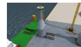
Onshore transfer of suction-type foundation
