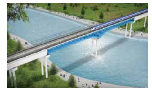
New-type of concrete Filled Tube Railroad Bridge
