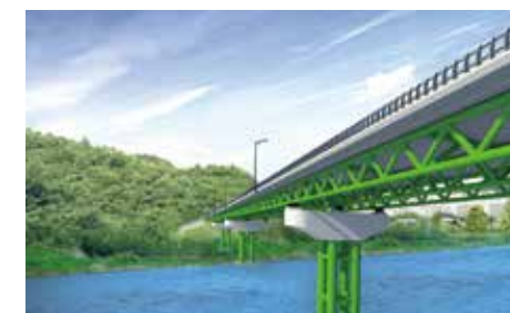
Concrete Filled Tube Highway Bridge + Modular Pier System
