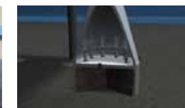
Underwater installation of suction-type foundation
