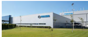
28 Mazda de Mexico Vehicle Operation Location: Guanajuato, Mexico Production capacity: 250,000 units per year Models in production: Mazda2, Mazda3, Compact vehicles for Toyota
