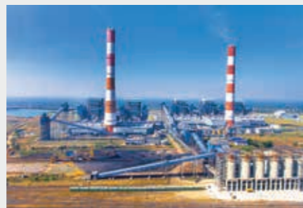
Adani Power Maharashtra Limited (APML)
