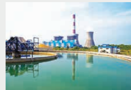
Udupi Power Corporation Limited (UPCL)
