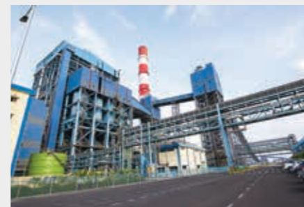
Adani Power Rajasthan Limited (APRL)
